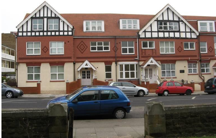
New development on Eastern Esplanade fits in well with the surrounding historic buildings
